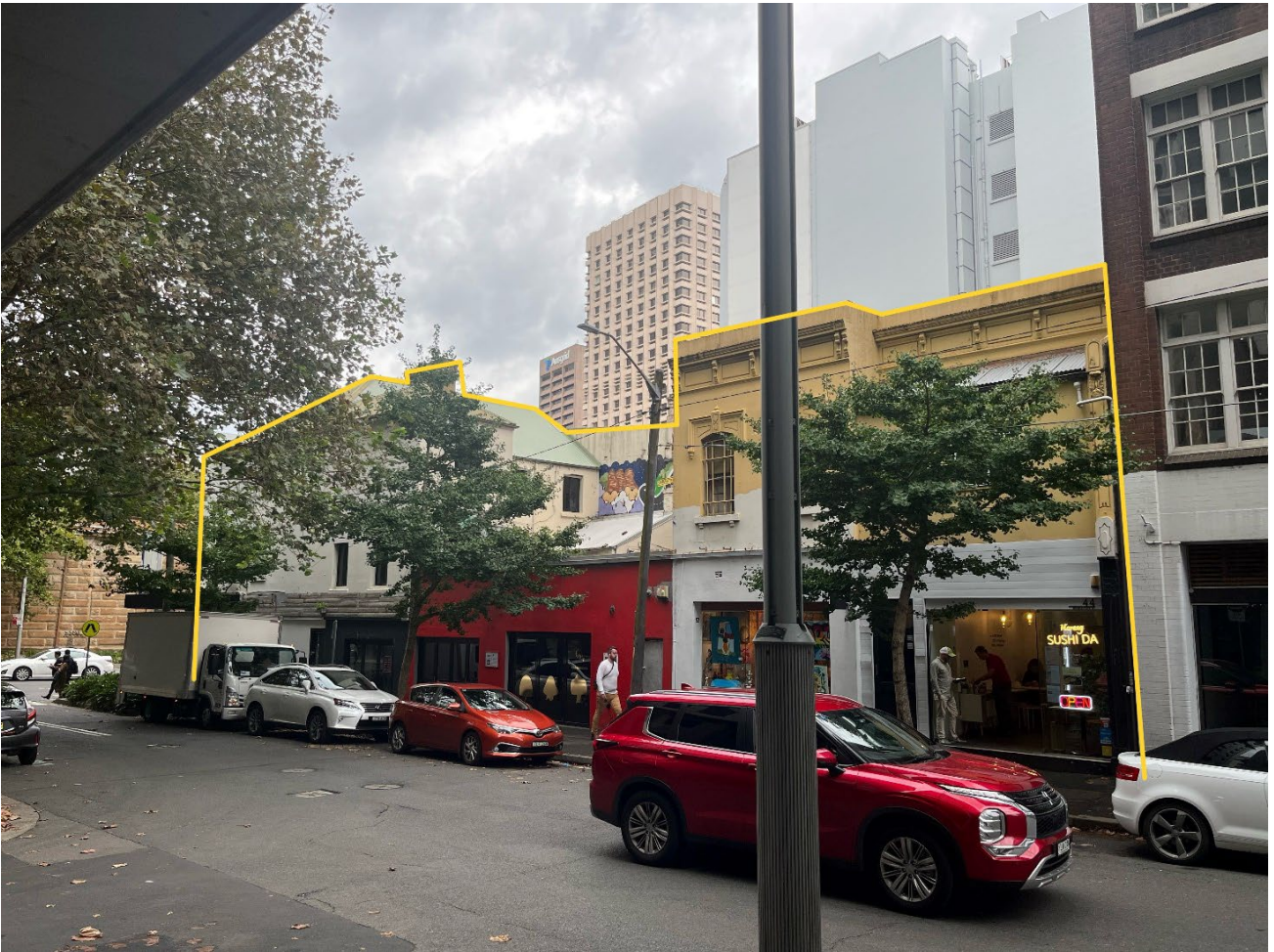
Figure 6. 232-240 Elizabeth Street, viewed from the south-east, outlined in yellow (Reservoir Street frontage)
